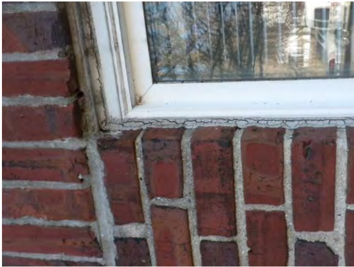
Example of the cracked/deteriorating window caulking
