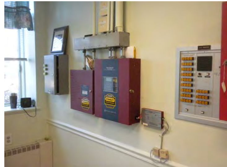
The central fire alarm control panel
