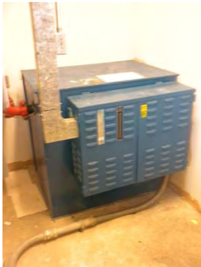
The hydraulic elevator equipment
