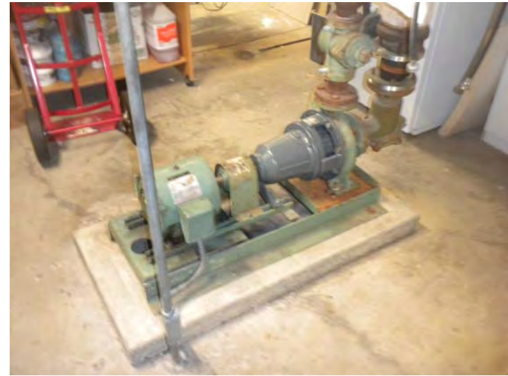
View of a re-built heating water pump (one of two)
