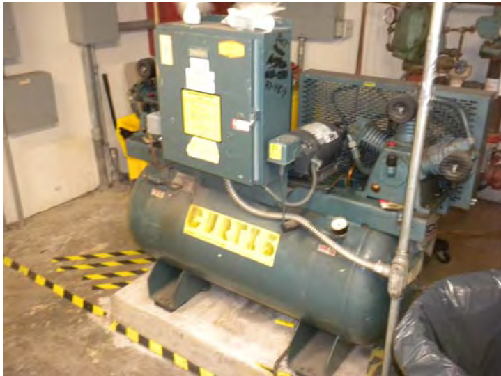
Pneumatic thermostat compressor
